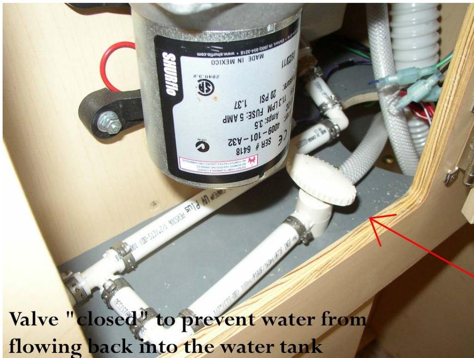
Valve "closed" to prevent water from flowing back into the water tank
