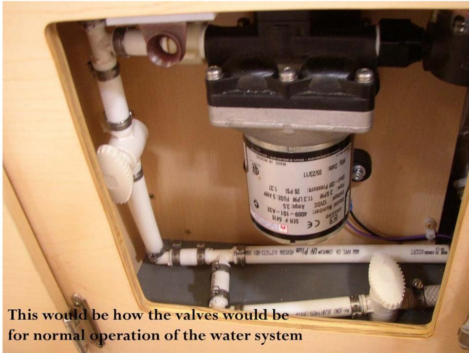
This would be how the valves would be for normal operation of the water system
